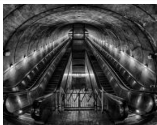
Class A - 1st Place Mike Jeffries - Rosslyn Escalators
